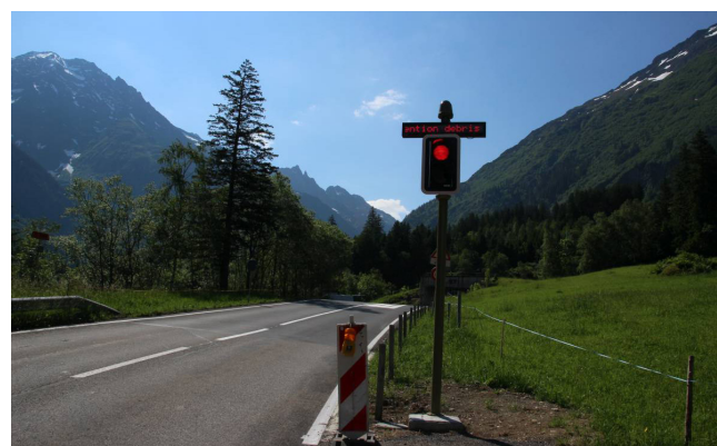
Figure 3: Several traffic light automatically close the road in case of an event. Further information on the closure reason is displayed for the waiting motorists.
